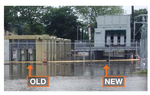
More than 4,600 PSE&G customers in Ewing and Trenton had power in May thanks to Energy Strong. The program built a new, elevated station (on right) that did not flood while the lower old station (on left) flooded on May 27, 2018 after storms. When completed 490,000 of PSE&G's 2 million customers who lost power during Sandy won't lose power again due to flooding.
